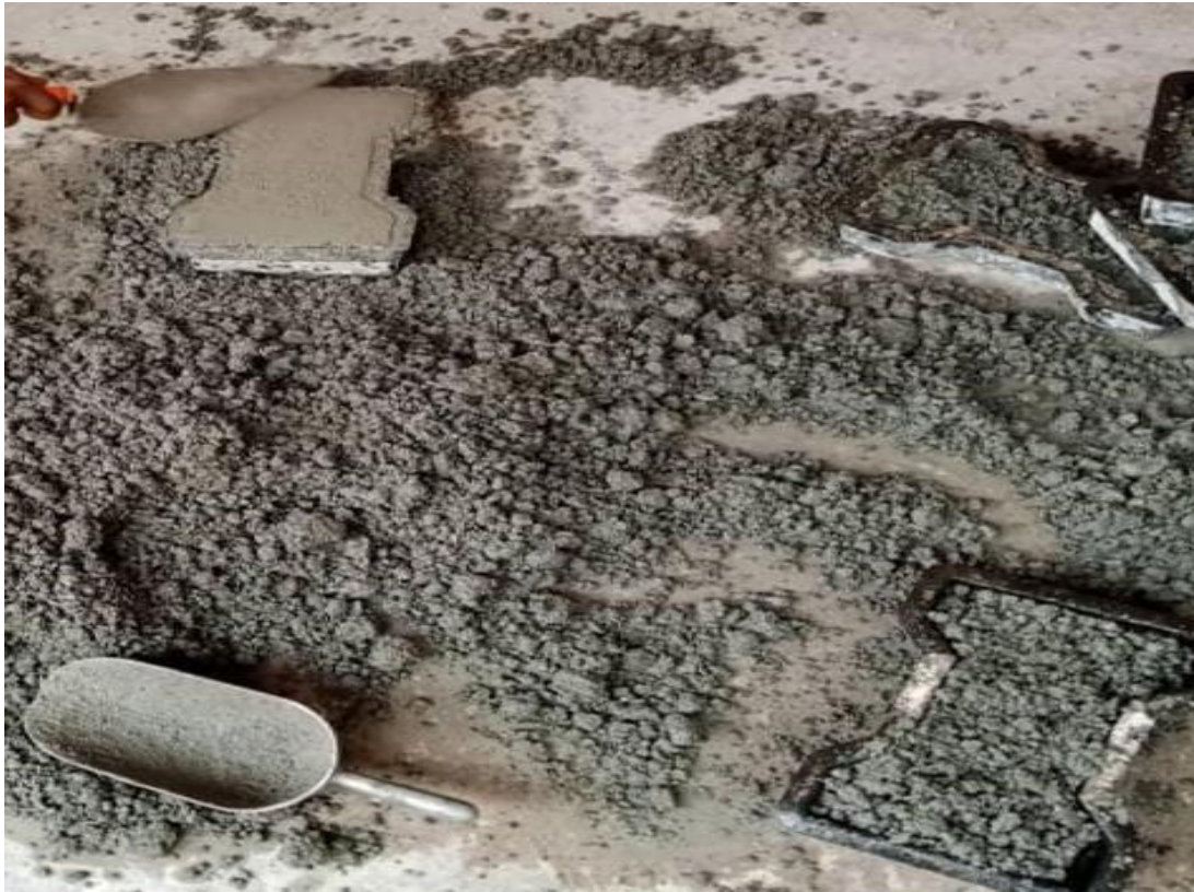
Figure 1: Casting of the Interlocking Tiles
