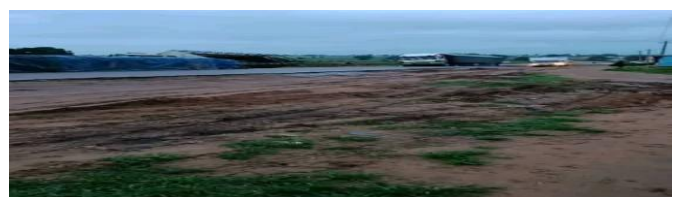
Absence of drainage (Keffi urban area)
